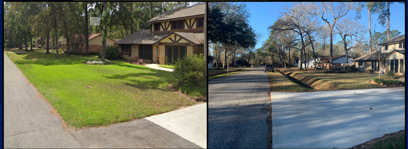
Midlothian Lane – Roadside Ditch
