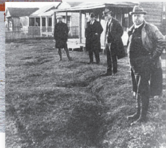
Earth fissures at Goose Creek Oil Field
